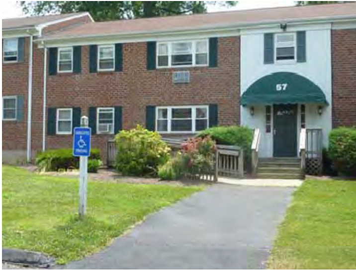
Repair and paint ramp to designated accessible unit 57-B.
