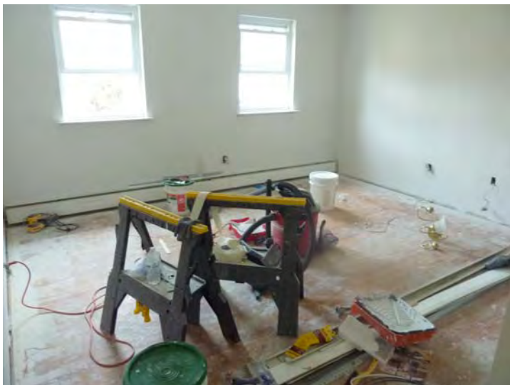
New hot water baseboards are being installed in apartment 53-B.
