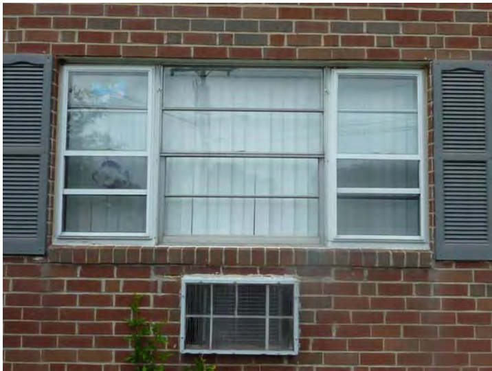
Original center double hung sash and more recent replacement flankers. Replacement of all co-op unit windows is shown in Year 1 based on EUL and condition.
